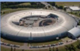
A synchrotron is a large ring structure, half a kilometre around, which accelerates a beam of electrons to almost the speed of light. As the electron beam is bent by large magnets, it creates bursts of energy in the form of X-rays, which can be directed towards the tissue samples.
